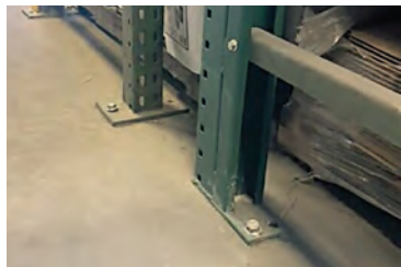
Typical low-corrosive environment — interior warehouse.
