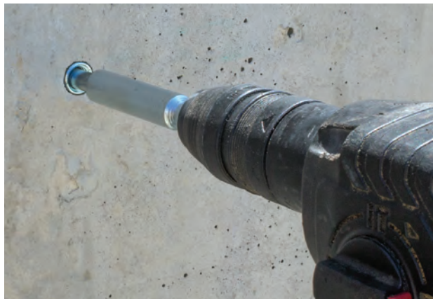
Anchor being set with SDS setting tool.
