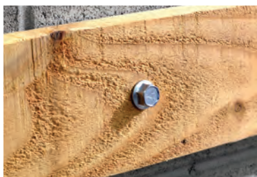
Anchoring adhesives, Titen HD (interior only unless using a stainless-steel version of the anchor), Strong-Bolt 2, Wedge-All
