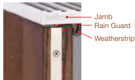
Top of door; exterior view.
